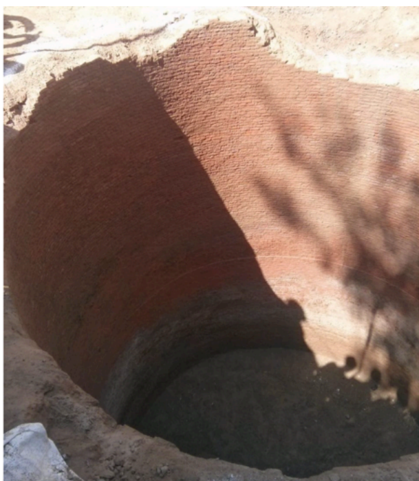
Figure 1. Abandoned well unearthed beneath a religious structure at Ajnala
