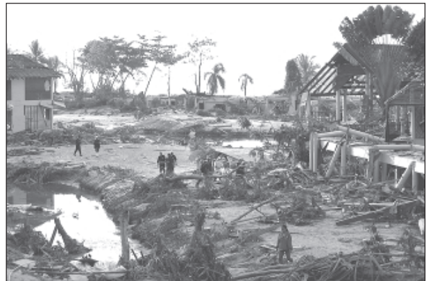
Fig 1: Destruction on the coast road to Takua Pa
